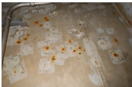
Typical crew repairs to a tank top after 6 months service
