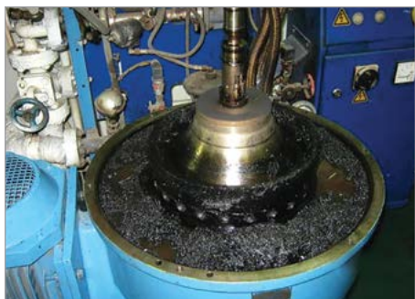
Sludge build-up in purifier. Image courtesy of Braemar Salvage Association
