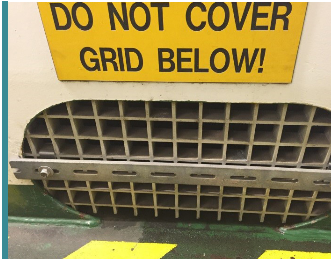
Fig 8: Vehicle deck drain
