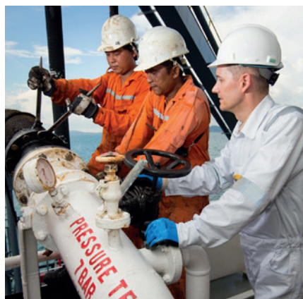
Fig. 7. The use of correct personal protective equipment is an essential part of shipboard bunkering procedures (VPS)
