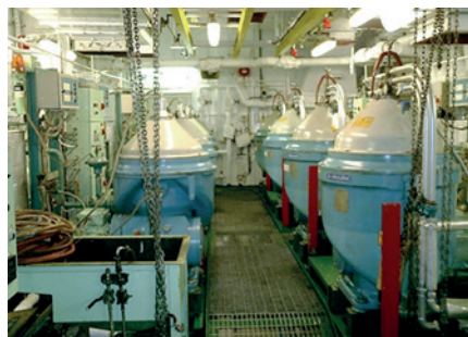
Fig. 26. Centrifugal separators on board a vessel
