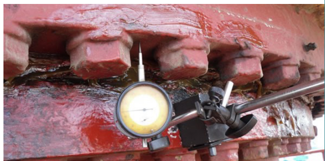
Example of examination with depth gauge and clock gauge
