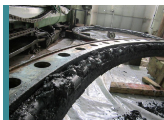
Rollers retaining ring damaged, rollers displaced.
