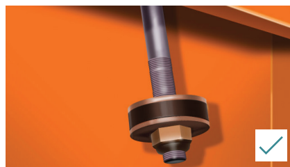
Cleat - washer in good condition
