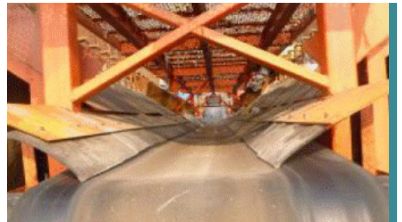
Overview of conveyor and steel mesh
