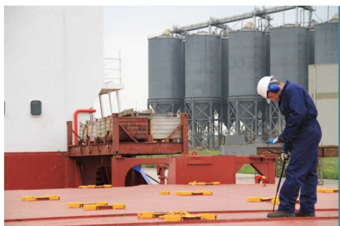
Ultrasonic hatch cover testing
