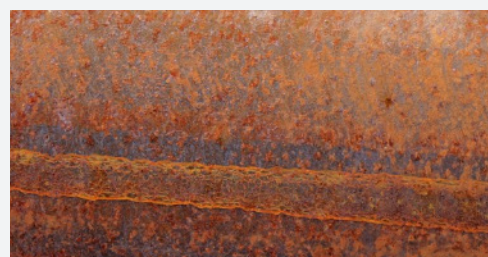
Example of oxidisation rust which would not affect the cargo
