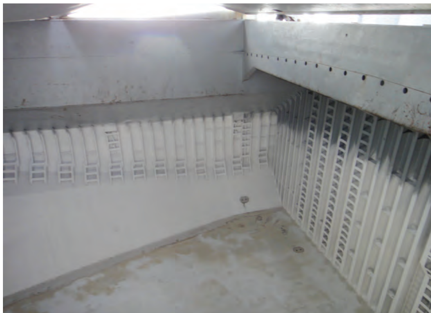
Fig. 13. The lime wash finished and drying, including the tank top
