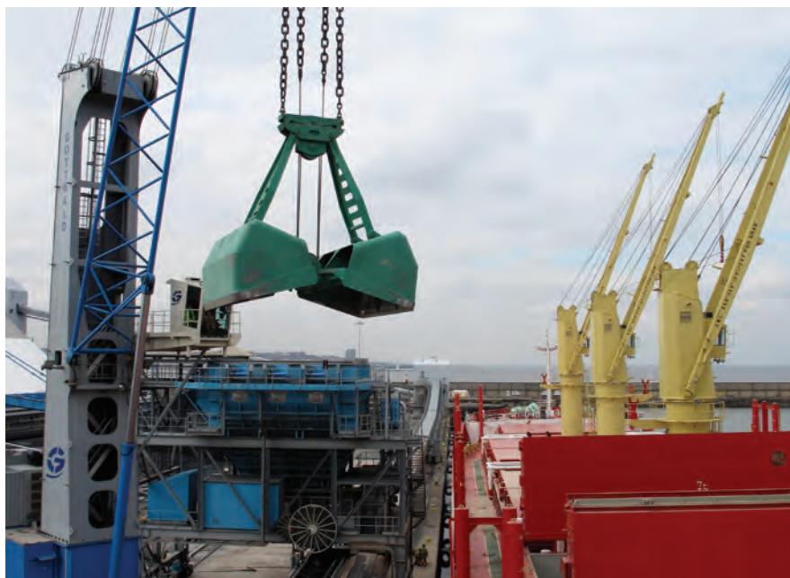
Fig. 19. Discharge by grab to an on-shore hopper
