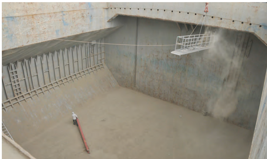
Fig. 31. The residues remaining after unloading cement
