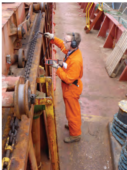
Fig. 4. Ultrasonic testing of hatch covers
