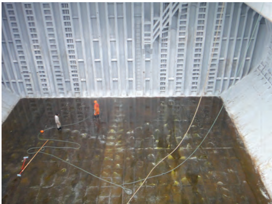
Fig. 12. Lime washing in progress, the tank top still to be done
