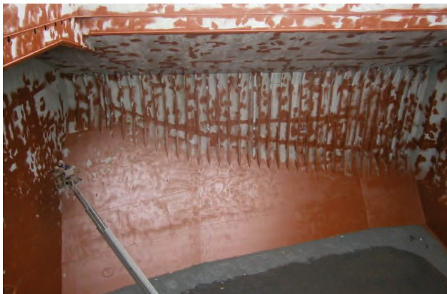
Fig. 15. Touch-up painting being undertaken
