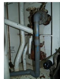
A magic pipe - in this case a temporary plastic pipe
